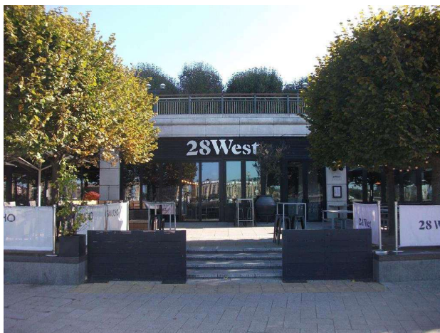
28 WEST FRONT VIEW
