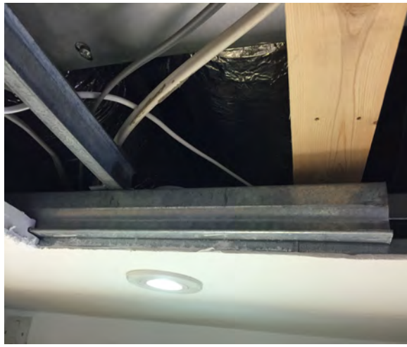
Photo 8: the metal frame where the slotted tile-side fits
