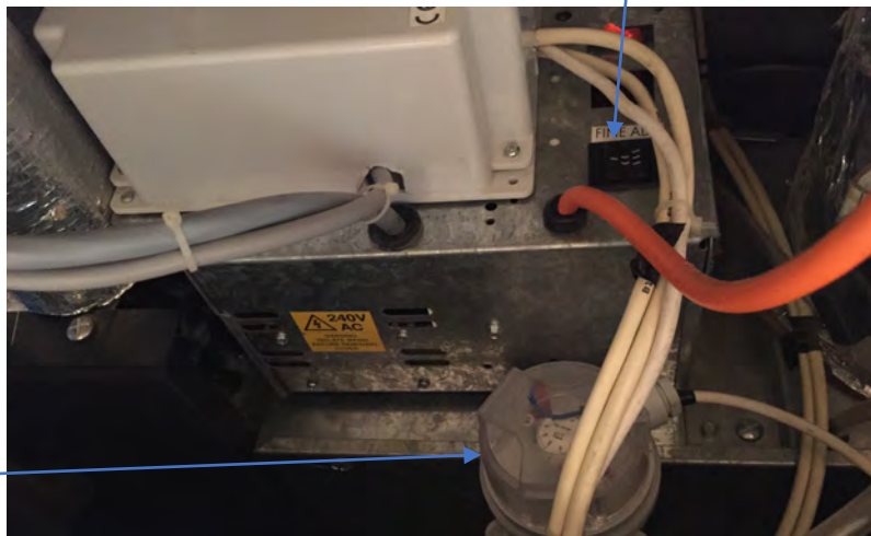
Photo 10: differential pressure switch and fan speed fine tuning
